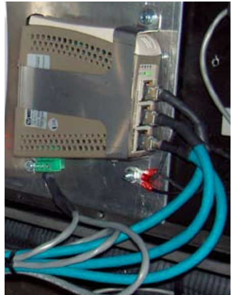
Westermo SDW-550B Ethernet switch in a Seattle bus
