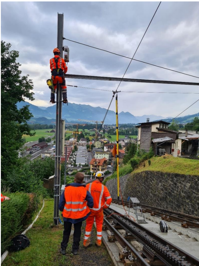
The Trackside Radio Equipment Box (TRE Box) being installed on Mount Pilatus
